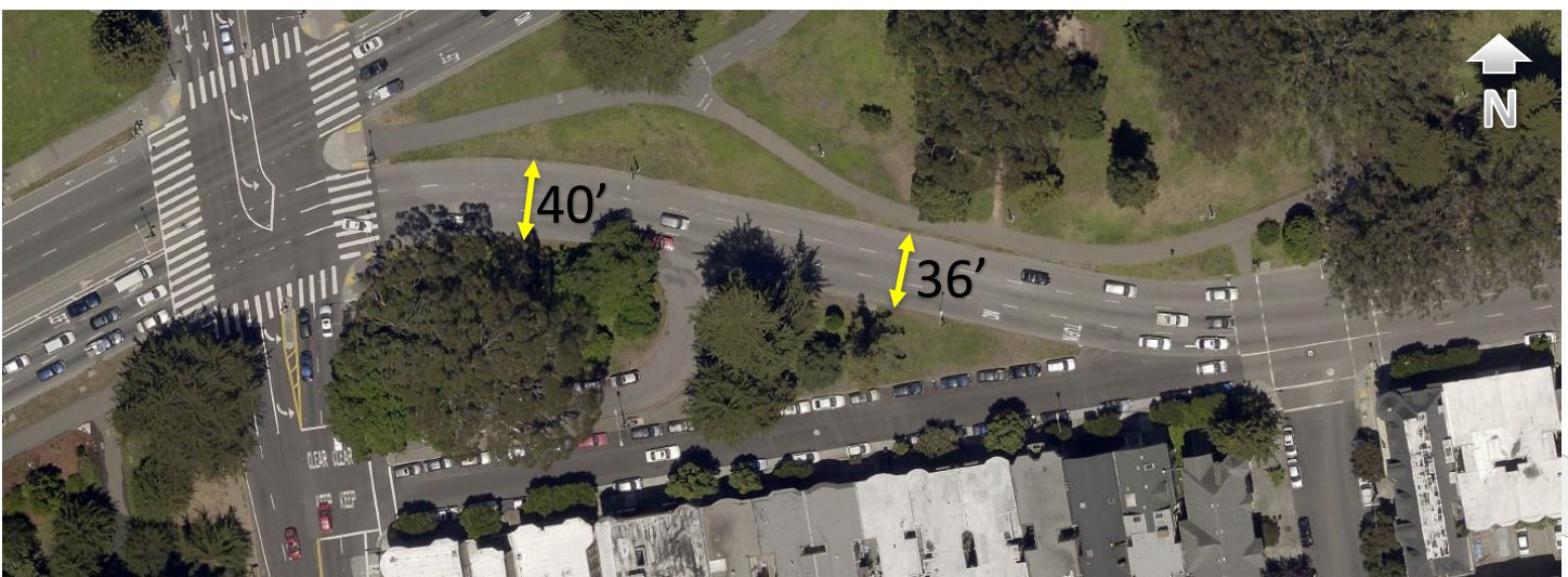
Figure 6 Aerial photo of Oak Street between Stanyan (left) and Shrader (right) streets, curb-to-curb width labeled
